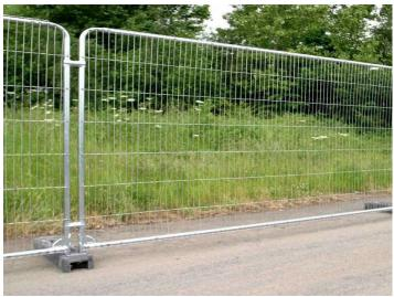
Photo 2 - Typical Heras Type Demountable Fence
