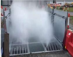
Figure 3.2e Example of static wheel wash systems
